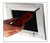
iv. Attach the frame wire with two dome head screws (provided with frame in a plastic bag). This will allow the frame assembly and back-box to be fastened securely together.
