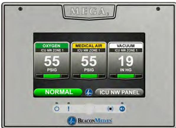
Figure 13: Area Alarm Front Panel
