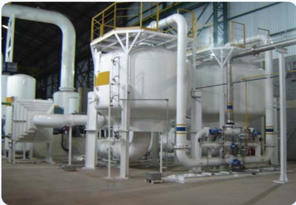
Two ASV80000 VPSA Oxygen Plants at a Steel Mill — Brazil
