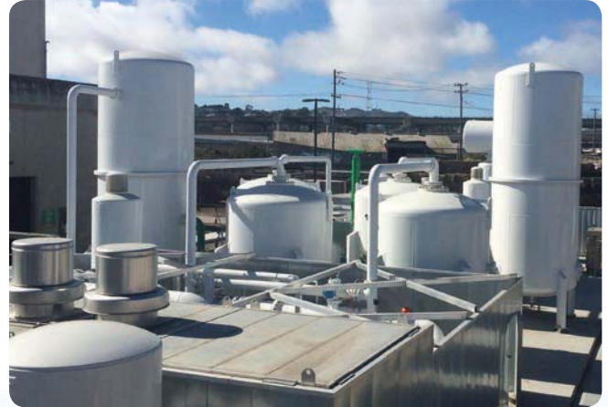
Two ASV45000 VPSA Oxygen Plants at a Wastewater Treatment Facility — San Francisco, CA USA
