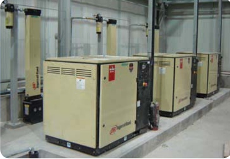
Instrument Air Compressor
