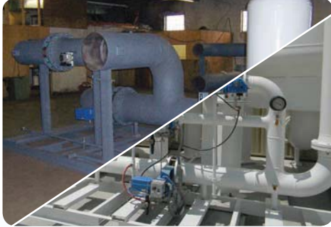
Feed & Waste Manifold and Product Manifold
