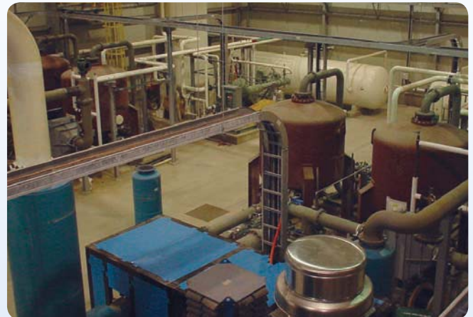
Two ASV25000 VPSA Oxygen Plants at a Uranium Mine — Canada
