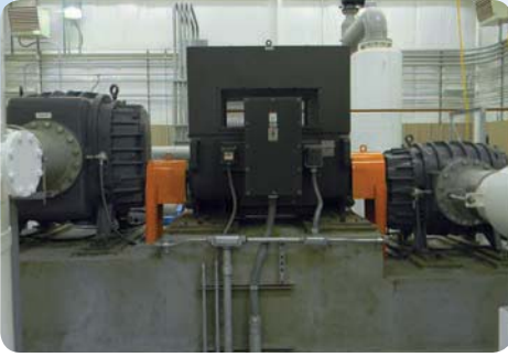
Blowers and Motor
