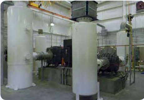
Inlet and Discharge Silencers
