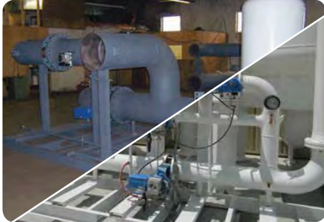
Feed & Waste Manifold and Product Manifold
