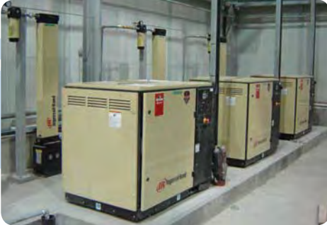
Instrument Air Compressor
