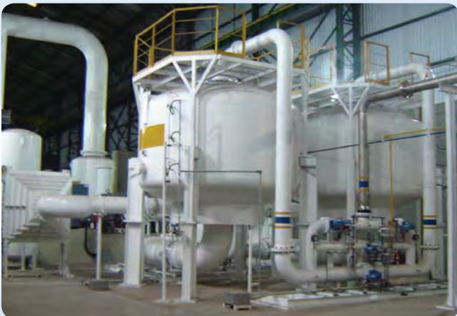
Two ASV80000 VPSA Oxygen Plants at a Steel Mill — Marabá, Brazil
