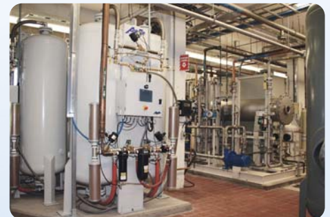
AS-L1000 Triplex PSA Oxygen Plant for ozone generation — St. Jean, Quebec, Canada
