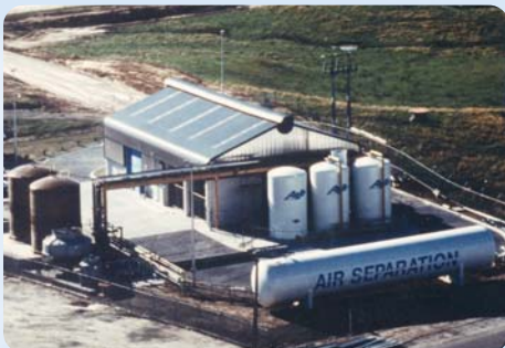
Installed and in operation at a Pulp and Paper Mill since 1991, this 42 TPD PSA Oxygen Plant supplies gas for bleaching and delignification.
