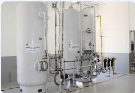
AS-Q2600-HM Duplex PSA Medical Oxygen Plant — Nicaragua
