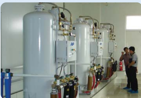
AS-K900-HM Triplex PSA Medical Oxygen Plant — China
