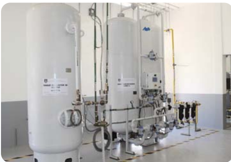
AS-Q2600-HM Duplex PSA Medical Oxygen Plant — Nicaragua
