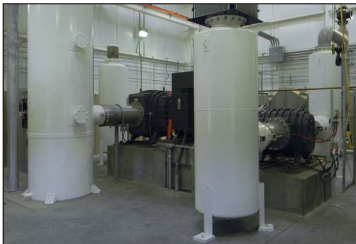
Silencers for vacuum blower discharge (left front), feed air intake (right front), vacuum blower suction inlet (left rear), and feed air blower discharge (right rear) complement user-friendly operator interface.
