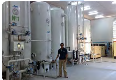
AS-Z5500-HM Duplex PSA Medical Oxygen Plant — Paraguay
