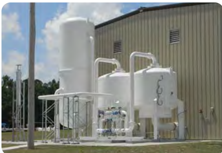
ASV27000 VPSA Oxygen Plant at a Wastewater Treatment Facility — Rocky Mount, NC USA
