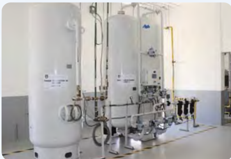
AS-Q2600-HM Duplex PSA Medical Oxygen Plant — Nicaragua
