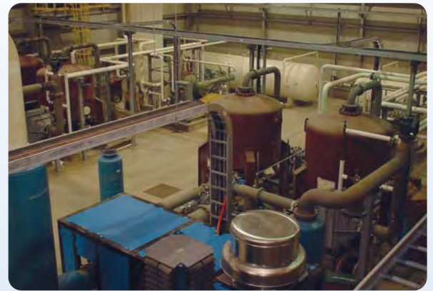
Two ASV25000 VPSA Oxygen Plant at a Uranium Mine — Canada
